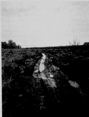
UNIMPROVED ROAD AFTER A STORM
